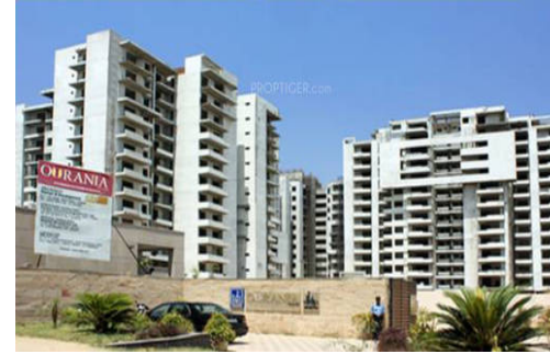
TDI Infrastructure Ourania Sector 53, Gurgaon
