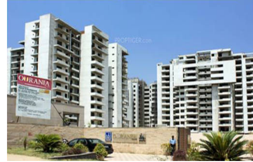
TDI Infrastructure Ourania Sector 53, Gurgaon
