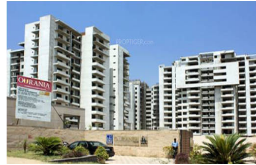
TDI Infrastructure Ourania Sector 53, Gurgaon
