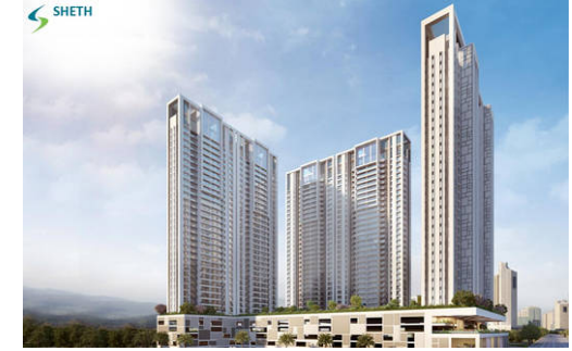
Sheth Corp Avante Kanjurmarg, Mumbai
