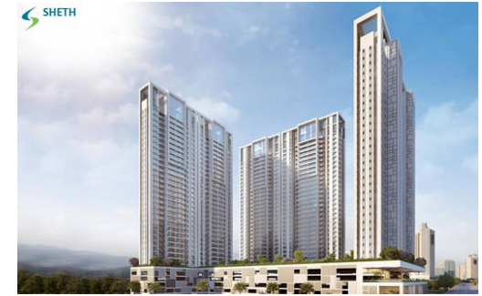
Sheth Corp Avante Kanjurmarg, Mumbai
