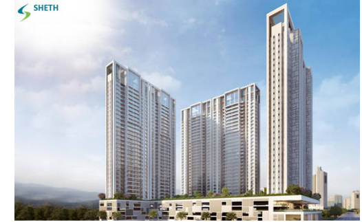
Sheth Corp Avante Kanjurmarg, Mumbai
