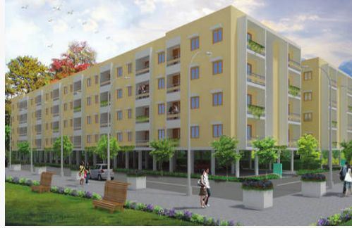
SSM Builders SSM Nagar Vandalur, Chennai
