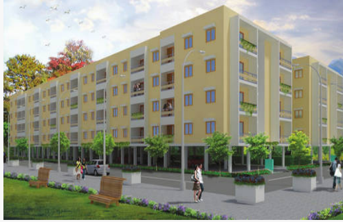
SSM Builders SSM Nagar Vandalur, Chennai
