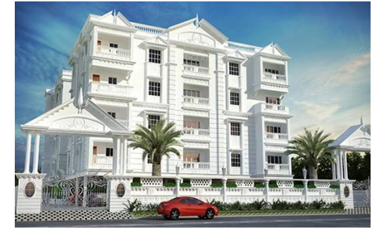
Rams Builders Anjali Atrium Nandanam, Chennai
