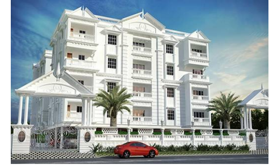
Rams Builders Anjali Atrium Nandanam, Chennai
