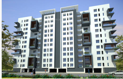
Appaswamy Greensville Sholinganallur, Chennai
