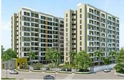
Nila Infrastructure Atuulyam Makarba, Ahmedabad
