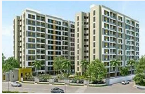
Nila Infrastructure Atuulyam Makarba, Ahmedabad
