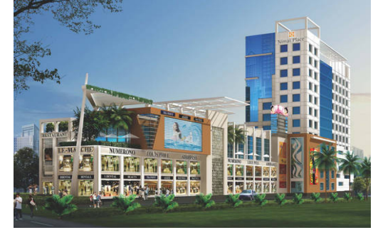
Nimai Place Sector 114, Gurgaon
